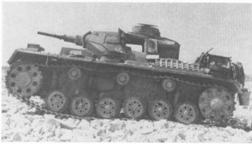
A Panzer III Ausf G of the Afrika Korps. Note the excellent accessibility provided by the turret side doors, and the characteristic pile of stores on the hull rear. (Imp. War Mus.)
