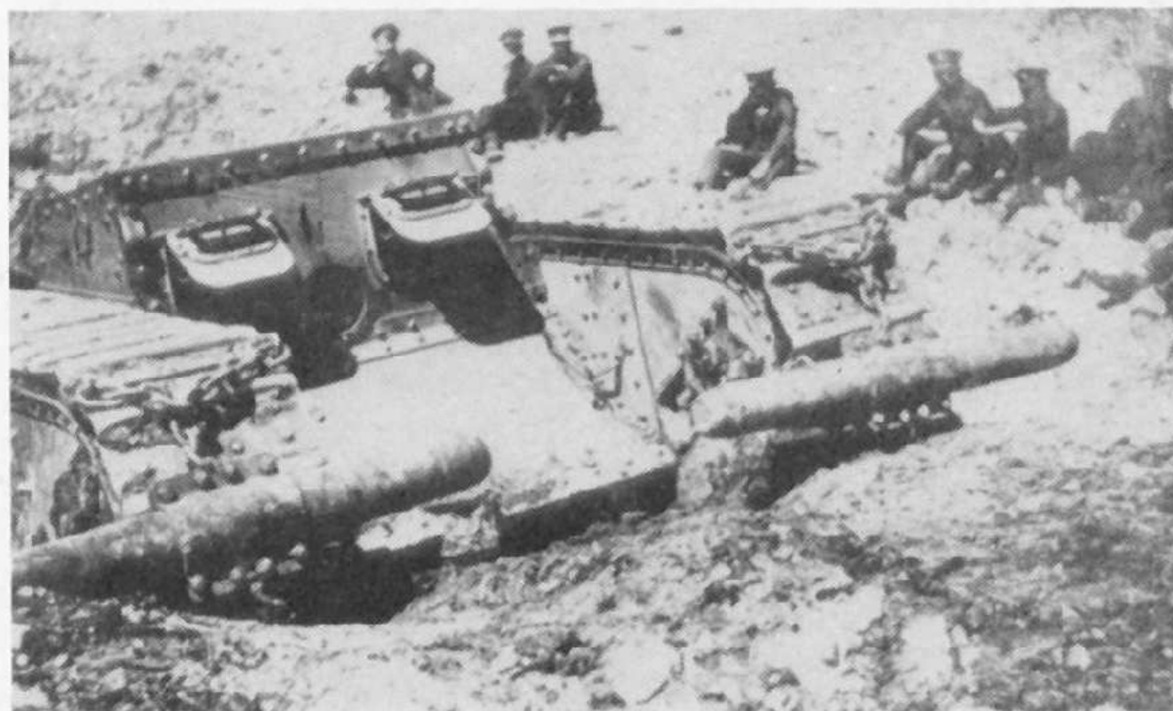
Prior to the introduction of the unditching beam torpedo spuds were used for the same purpose. Here tank crews under training watch a demonstration of their use. (Imperial War Museum)
