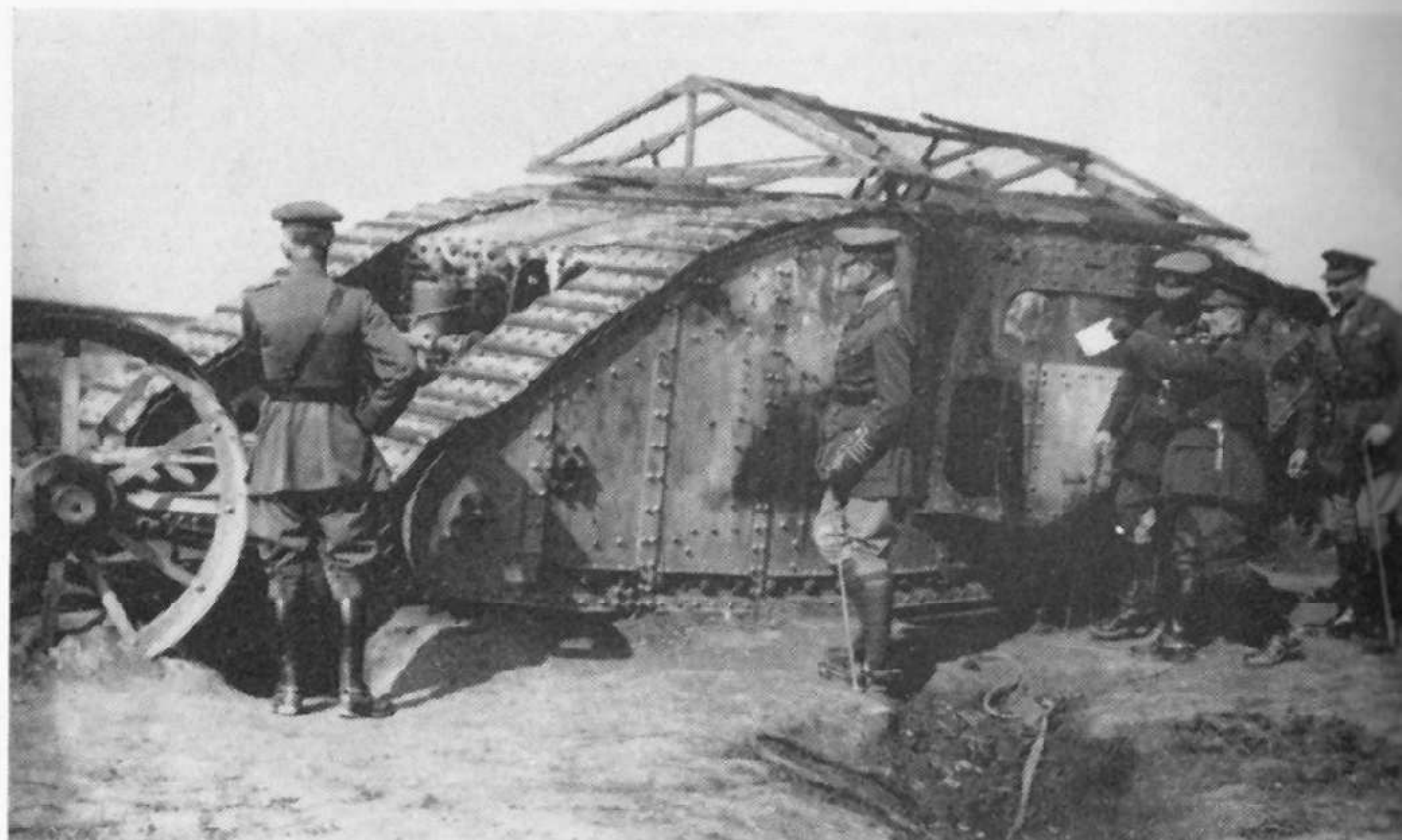
The King of the Belgians inspects a knocked out Mk. I after the Flers-Courcelette action. This is a female. Note the door in the sponson, the bomb roof and the "tail". (Imperial War Museum)
