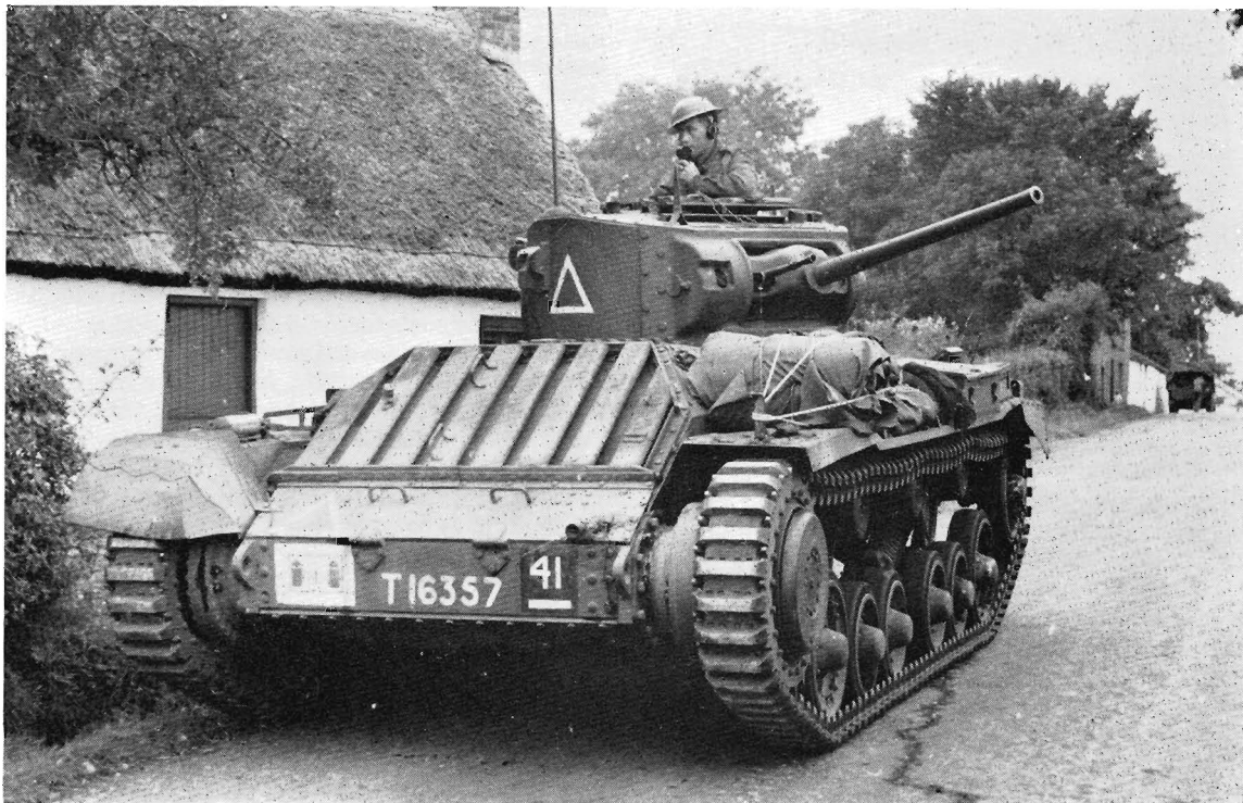
Valentine I with narrow tracks with a tread pattern like those of the Cruiser Mark III, IV, V and VI series. It was, however, of the twin guide horn type like other Valentines. The heavy armoured louvres on the rear deck show up well in this rear view. The formation sign on the left is of forces in Northern Ireland. (Imp. War Mus.)
