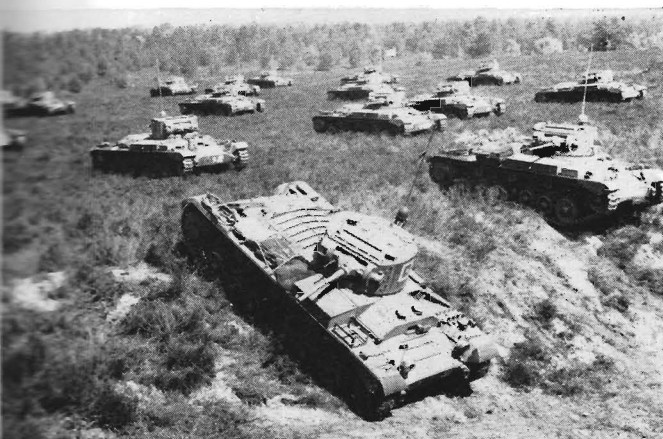
Valentine IIs of 48th Royal Tanks (21st Army Tank Brigade) on an exercise in Suffolk in June 1941. These tanks are fitted with the No. 11 wireless set, later superseded by the No. 19 set. The Brigade did not go into action with Valentines, but with Churchills (Infantry Tank Mk. IV), the first to do so—in Tunisia, 1943. (Imp. War Mus.)
