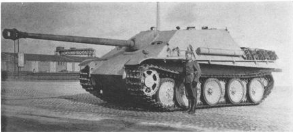
A very early production Jagdpanther (possibly, indeed, the prototype) showing the one-piece 8.8 cm. barrel which characterized early models. The unusual twin vision port for the driver supports the view that this is the prototype vehicle.
