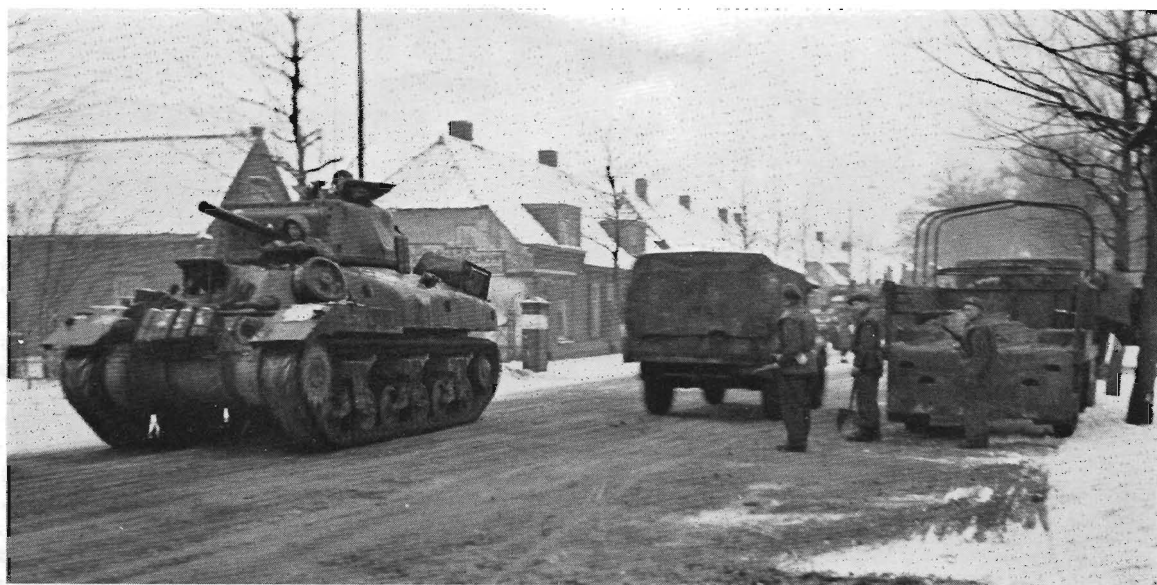
Ram OP tank of a Sexton-equipped SP field regiment passing through a village street in Holland in January 1945.
