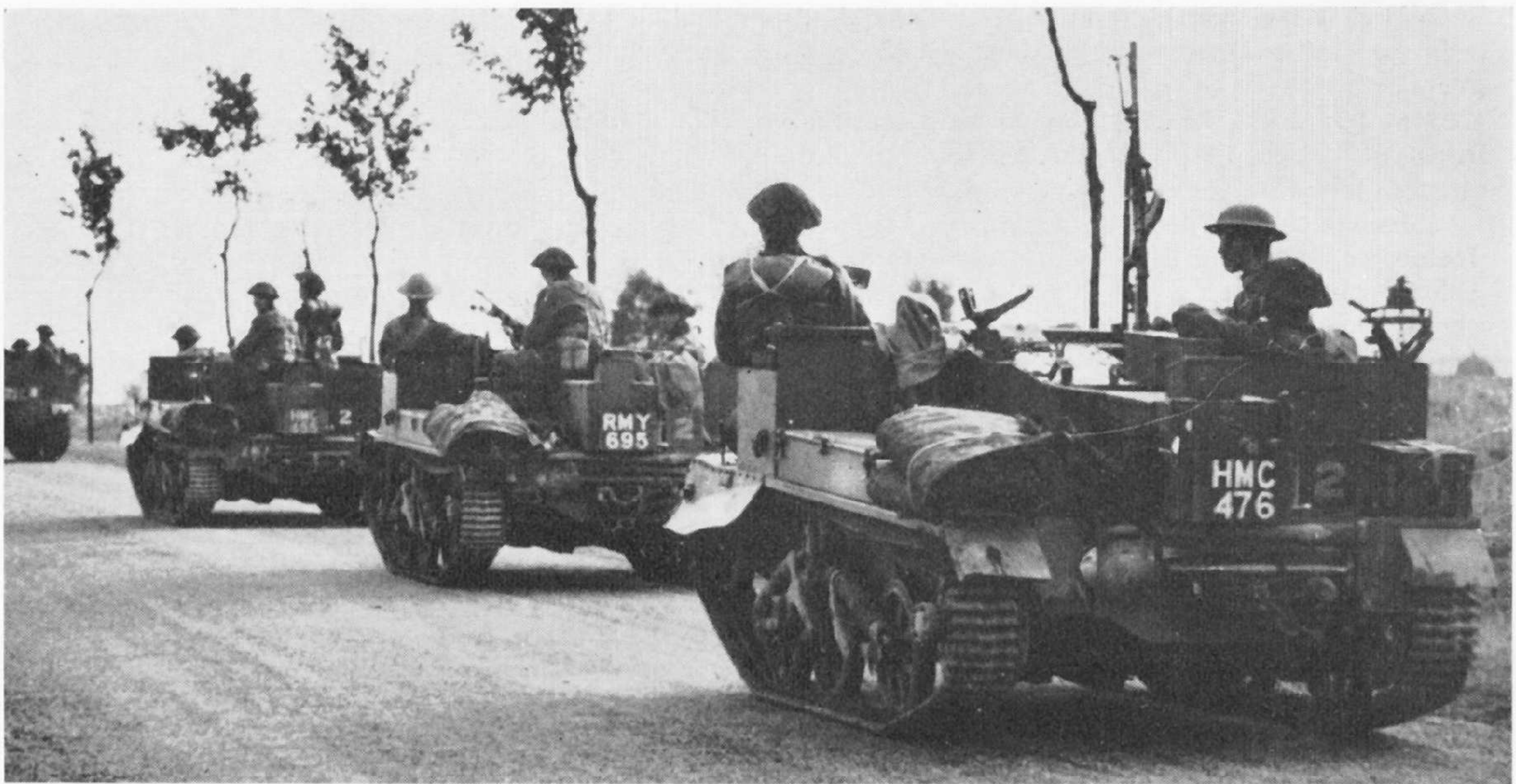
Scout Carriers of the British Expeditionary Force in France, September or October, 1939. Note left side open for stowage. Rear vehicle has base for wireless aerial fitted.
