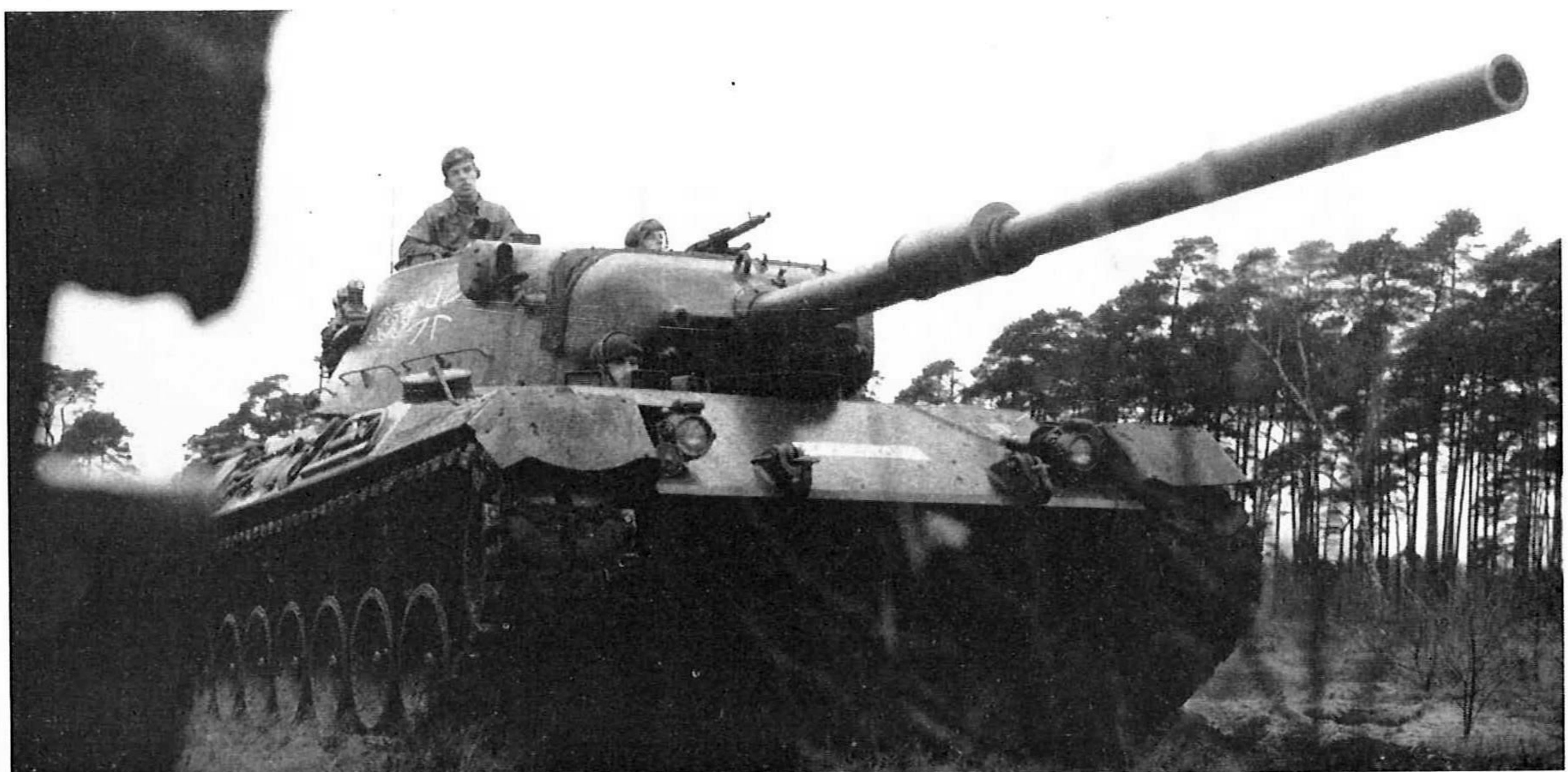
Leopard driver's three periscopes in front give a 130° arc of vision.
