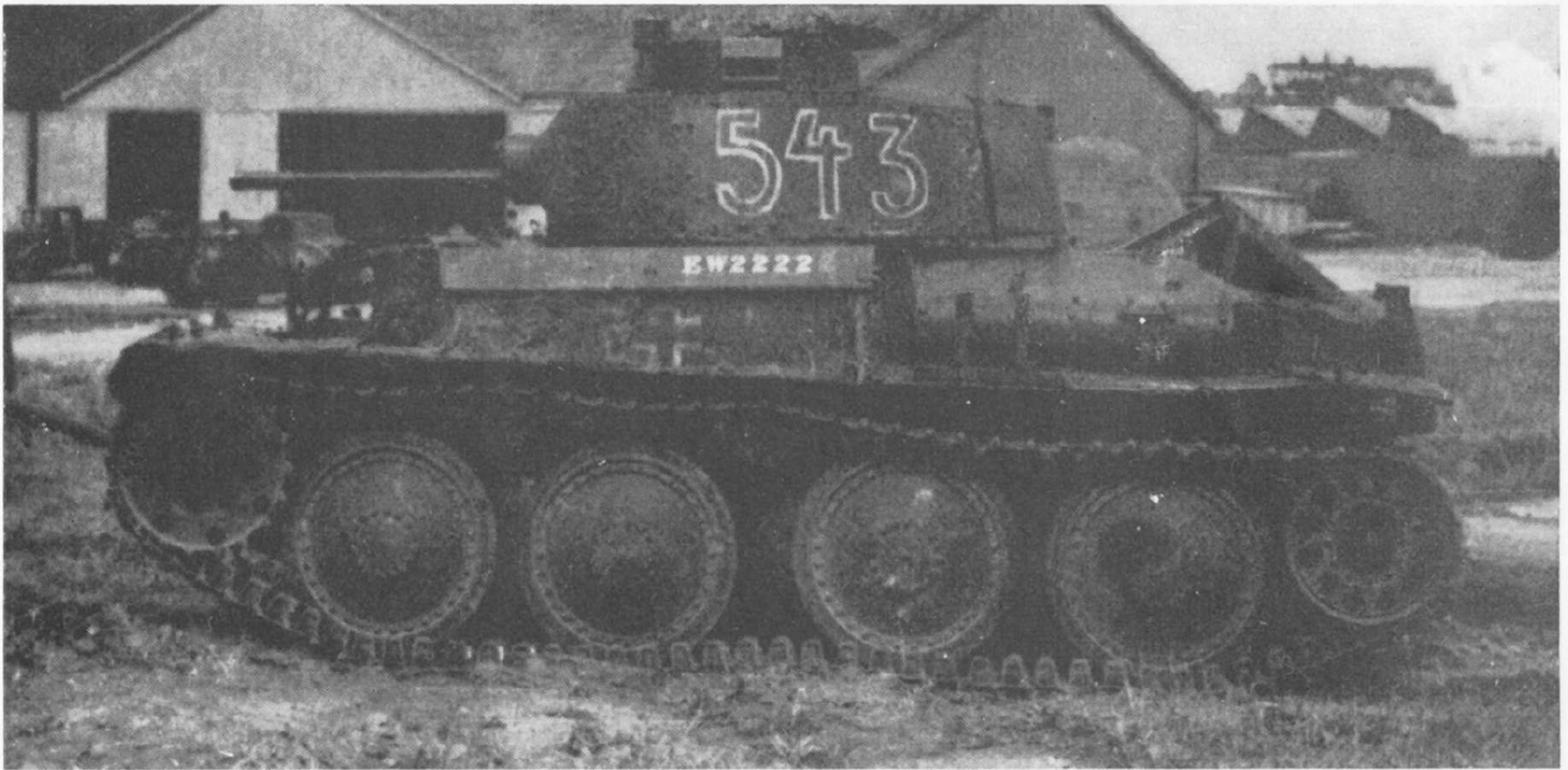
Above and below: Fifth production model TNHP (Model E) with new stowage arrangements (note the long stowage boxes placed along the sides) and internal modifications. (Milsom Collection)
