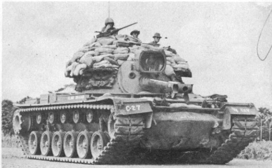
An M48A3 in South Vietnam with sandbags on the turret forming a bunker of sorts.
