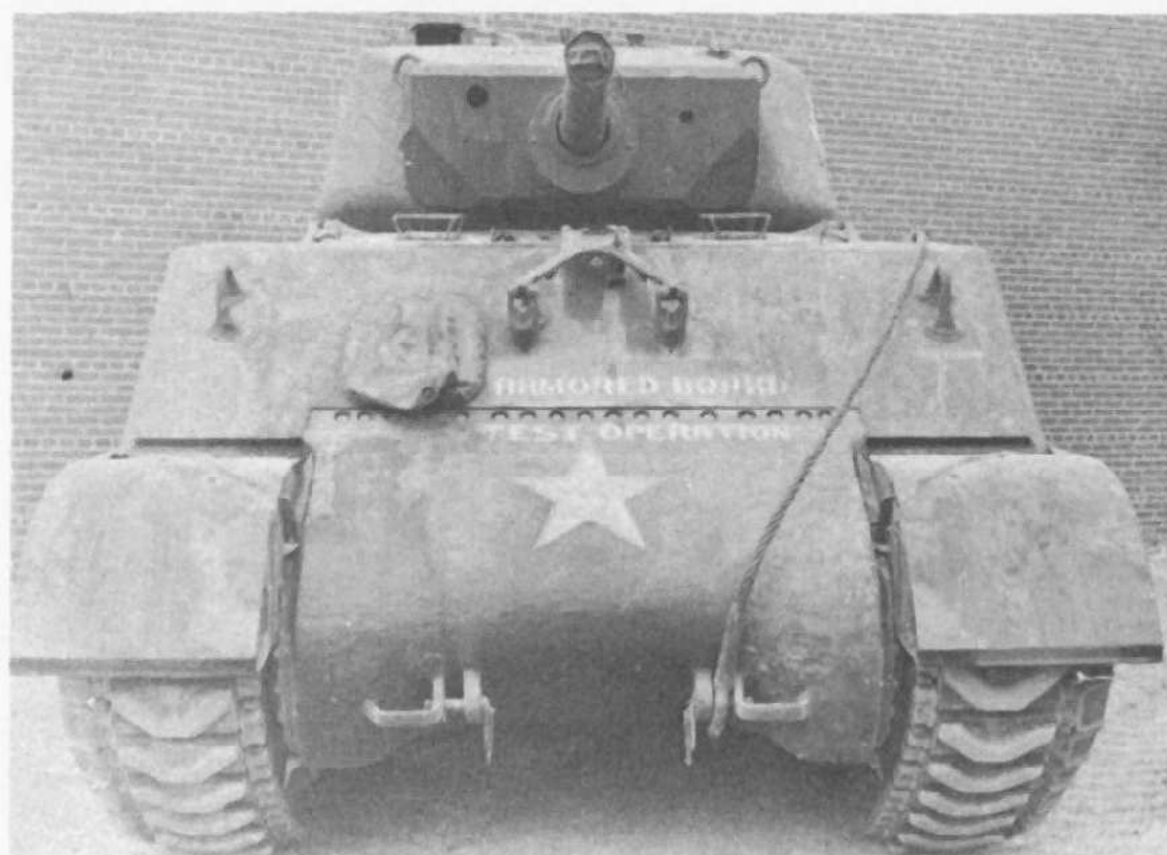
M4A3E2 "Jumbo" was a special assault tank built for the invasion of N.W. Europe to make good the American deficiency in heavy tanks. A new cast turret was made, plus a new heavy cast nose. Rest of hull was thickened with additional armor sheets, clearly visible in the front view. Grousers were a permanent fitting because of the extra weight.
