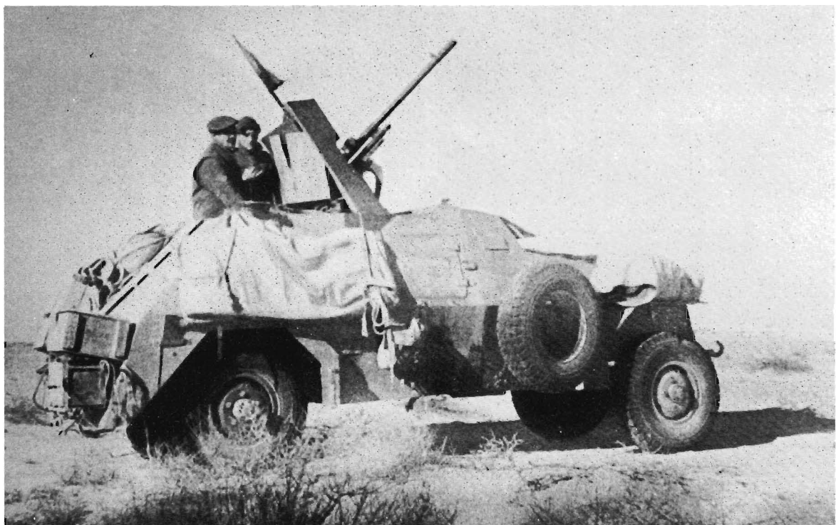
"Breda" car. Marmon-Herrington Mark II of The Royal Dragoons modified to take a captured Italian 20-mm. Breda gun. Unless a patrol was accompanied by a Breda car it had very little striking power. "It was generally supposed that the Boys anti-tank rifle . . . was unable to pierce any armour other than that of the Marmon-Herrington armoured car itself," wrote The Royals' regimental historian. (Photo: Major K. G. Balfour, M.C.)
