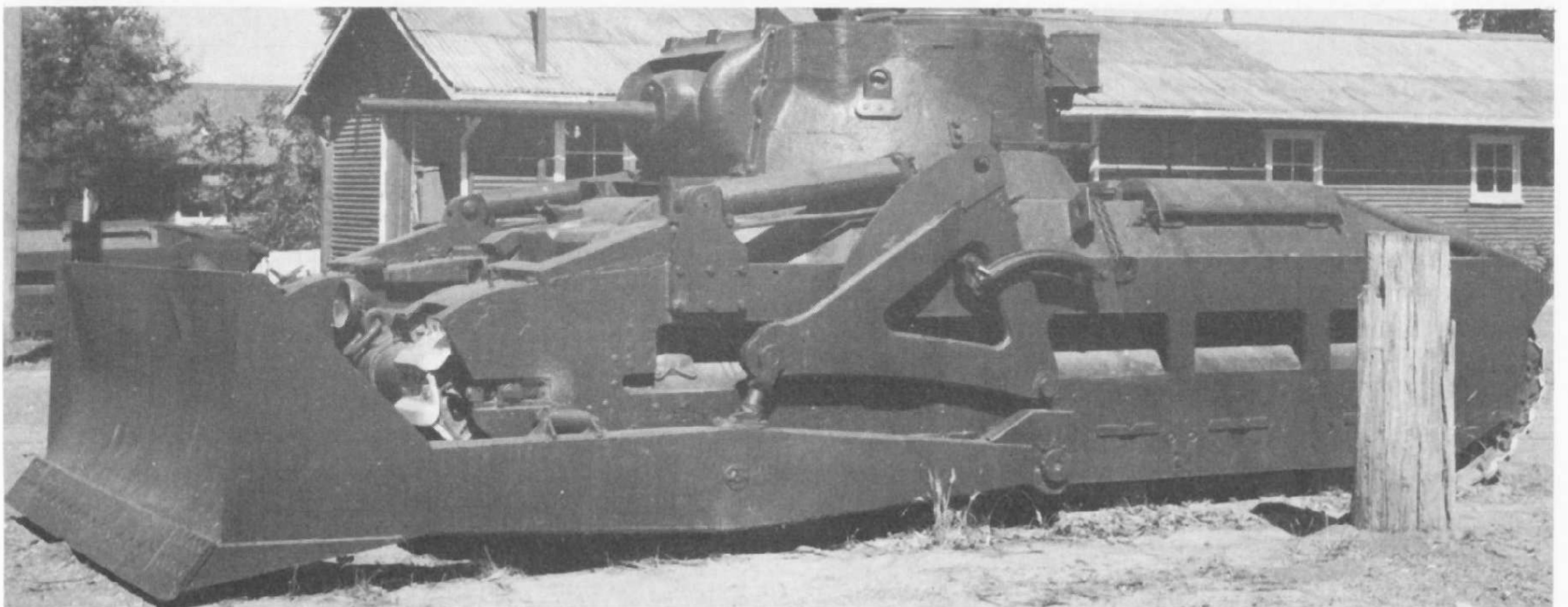
Australian Matilda Dozer No. 3. The blade and push poles could be jettisoned without exposing the crew, and the tank could then fight as a normal gun tank. (Photo: R.A.A.C. A.F.V. Museum)
