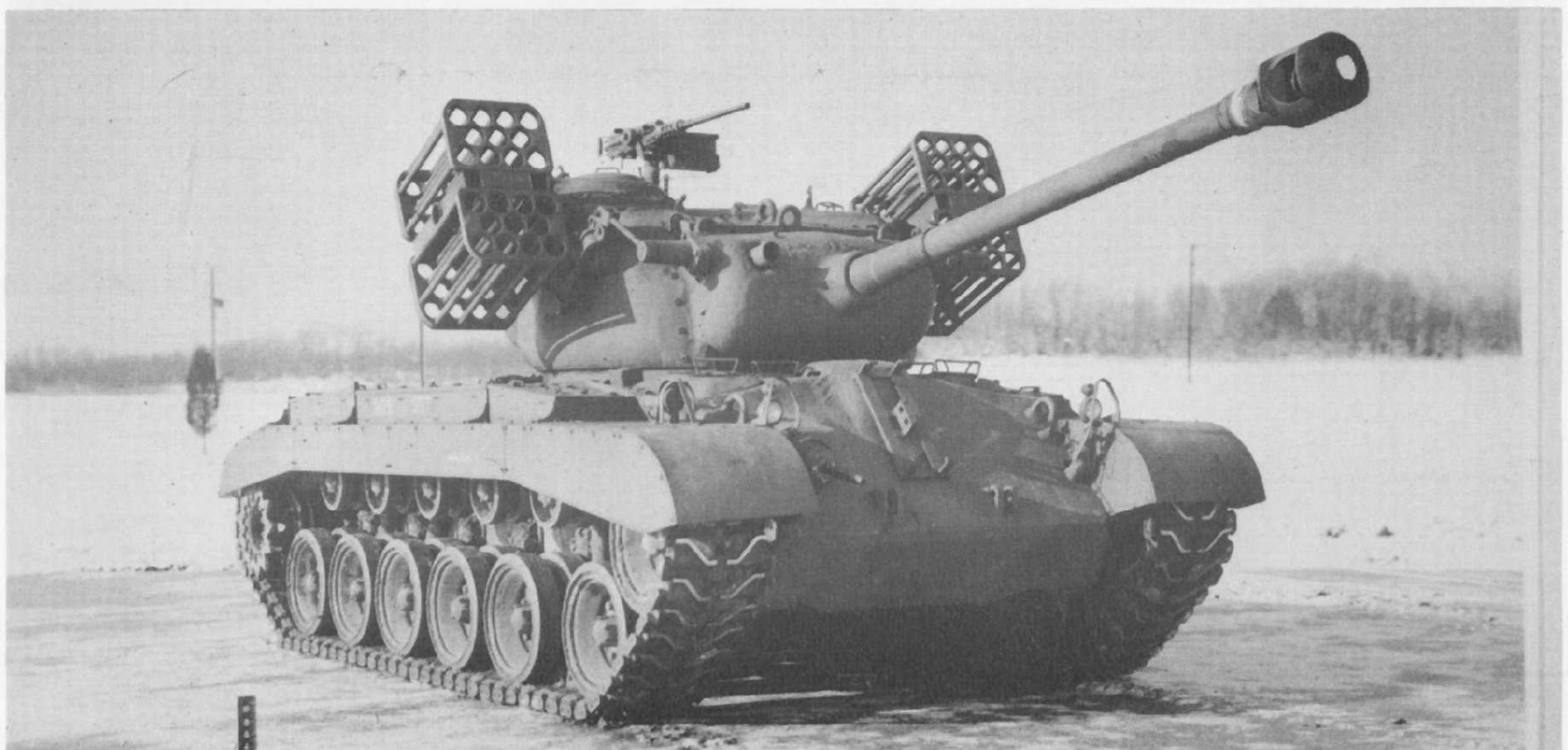
M26 Medium tank with experimentally mounted T99 Multiple Rocket Launcher.
