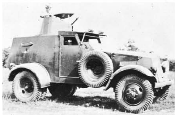
The T6 armored car was a re-built T7 car, but was no longer interchangeable with a truck body.
