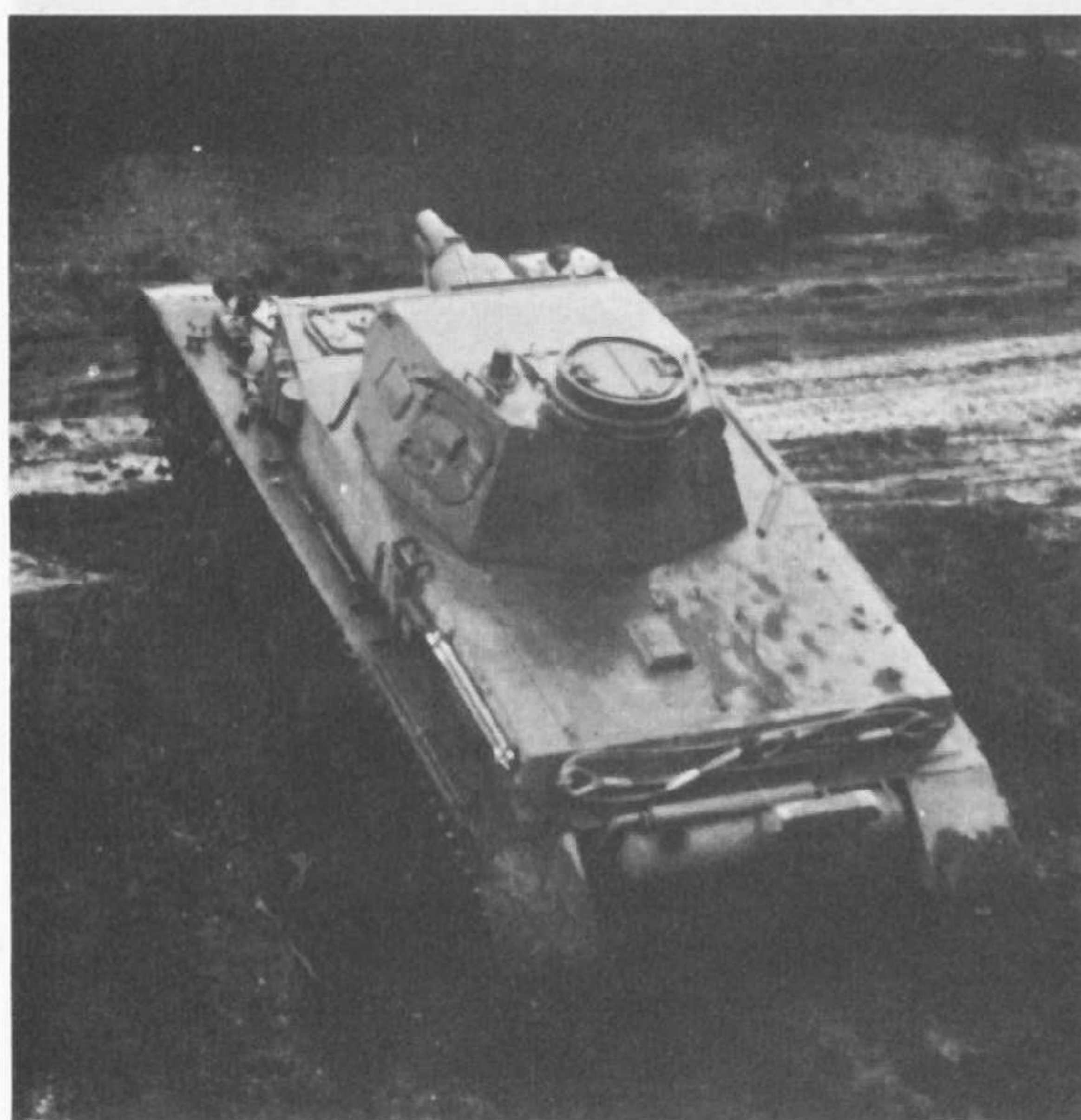
Three-quarter rear view of Ausf. D shows clearly the shape of the commander's cupola compared with that on Ausf. A. The four return rollers identify all Panzer IV vehicles.
