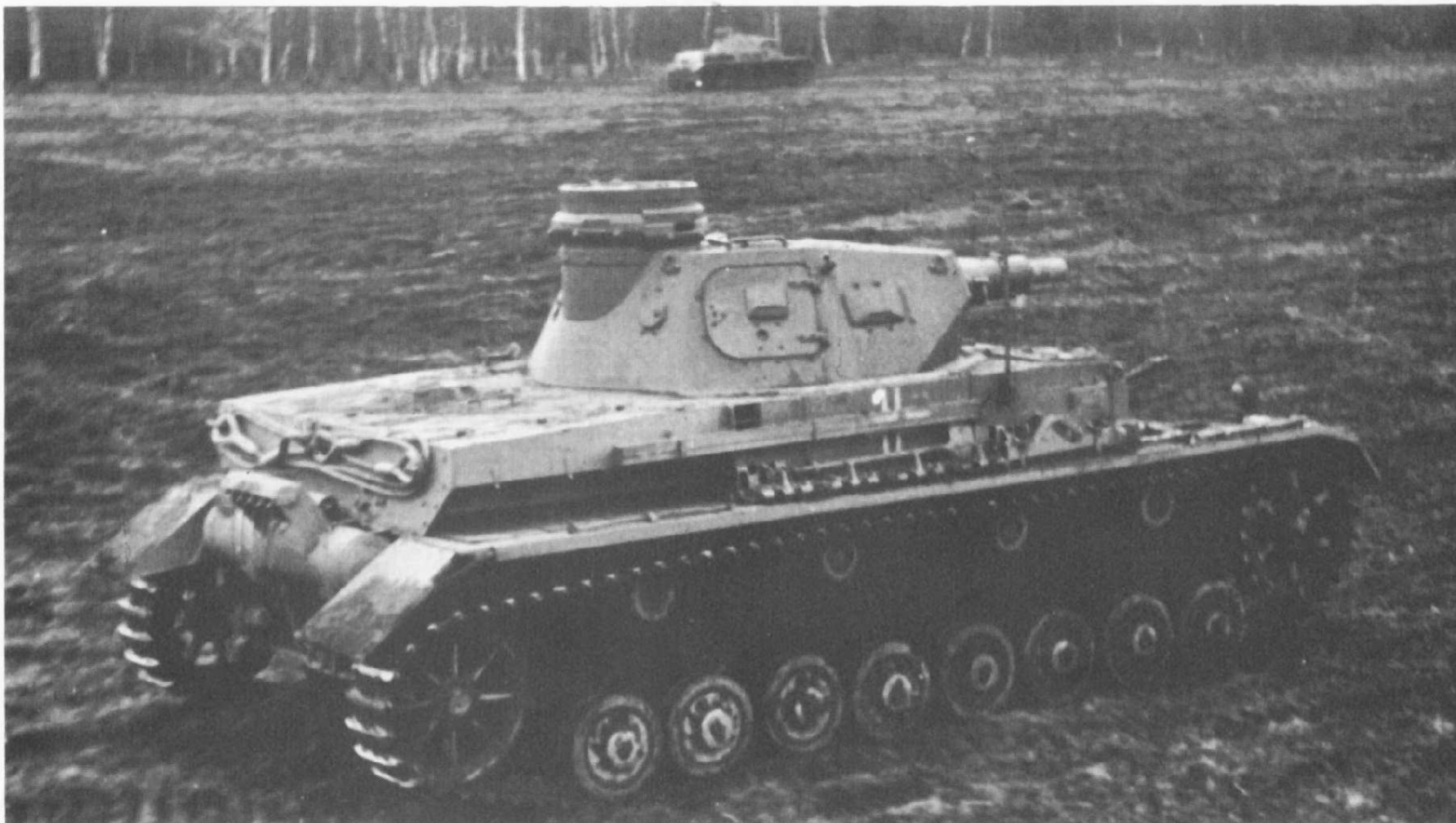
Three-quarter rear view of Ausf. D shows clearly the shape of the commander's cupola compared with that on Ausf. A. The four return rollers identify all Panzer IV vehicles.
