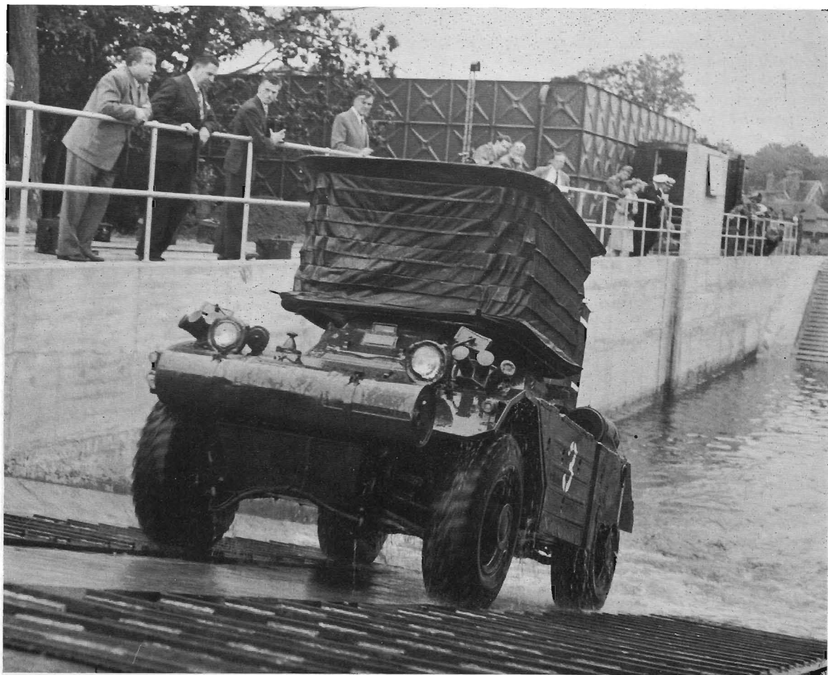
Ferret Mark 1 with deep wading equipment.
