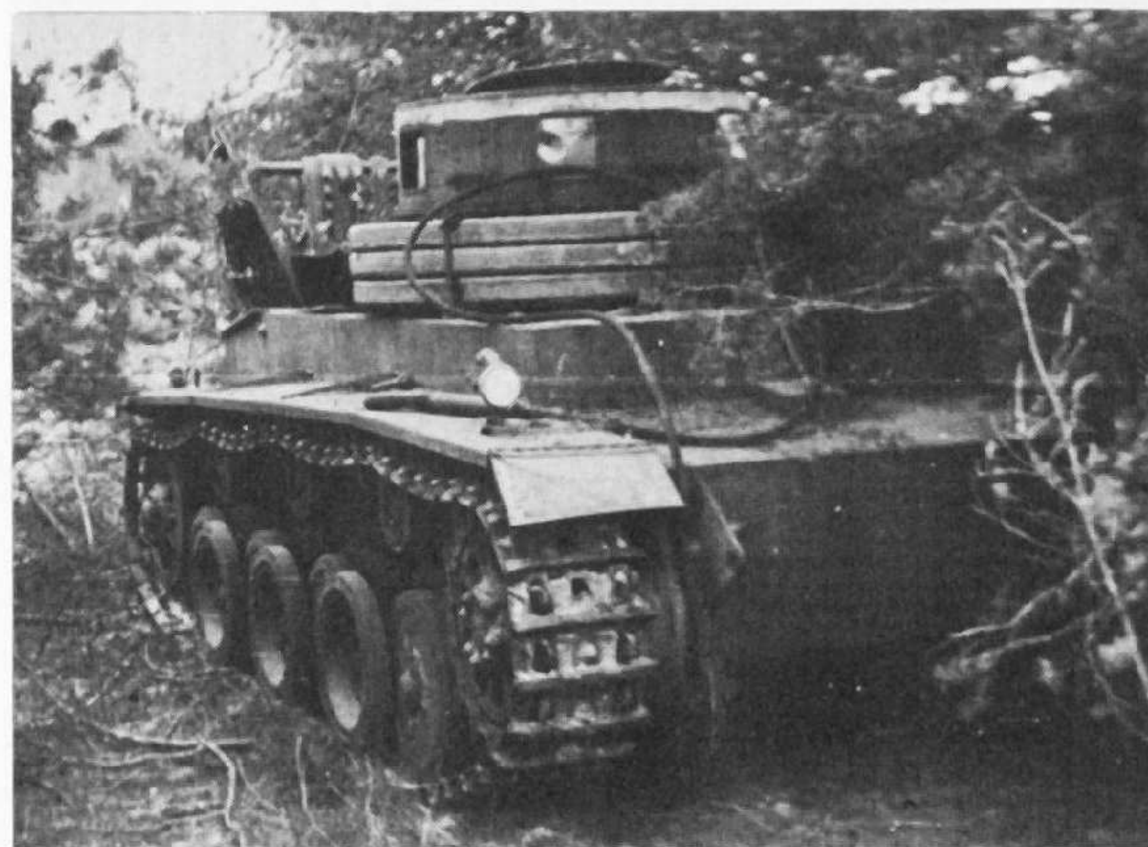
(Top right) Early progenitor of Henschel's Tiger Ausf. E (originally Ausf. H) was the 30-ton VK.3001 project. This is one of four prototypes built by Henschel in 1941. (Chamberlain Collection/Col. R. J. Icks)
