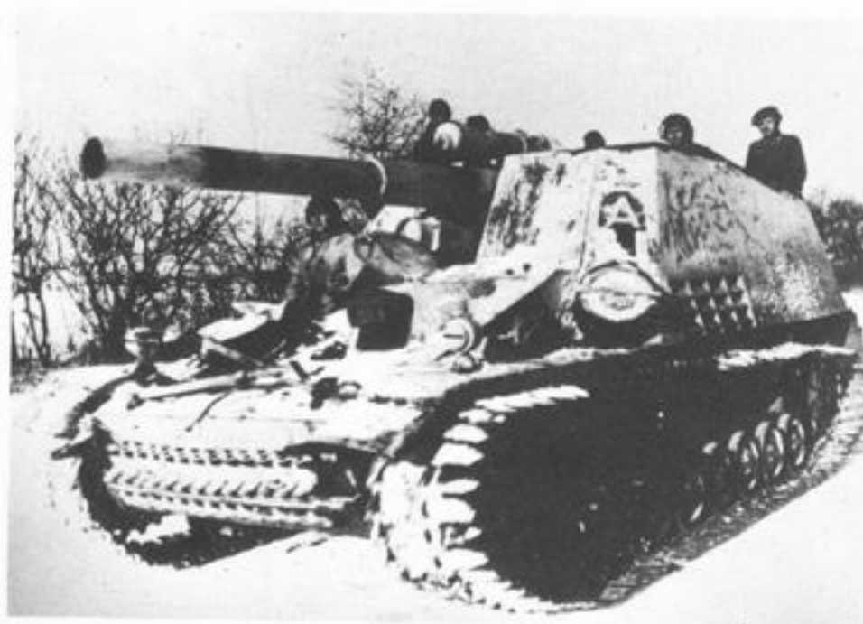
Hummel fitted with the Ostkette (East track). This was a lateral extension to the normal tracks for improved ground pressure and better traction over soft ground.
