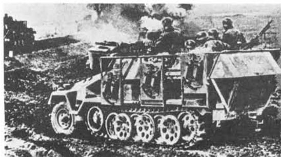
This SdKfz 251/1 shown here in Russia carried three frames on each side to mount either the 28 cm. high explosive or 32 cm. napalm rockets. (Spielberger Collection)
