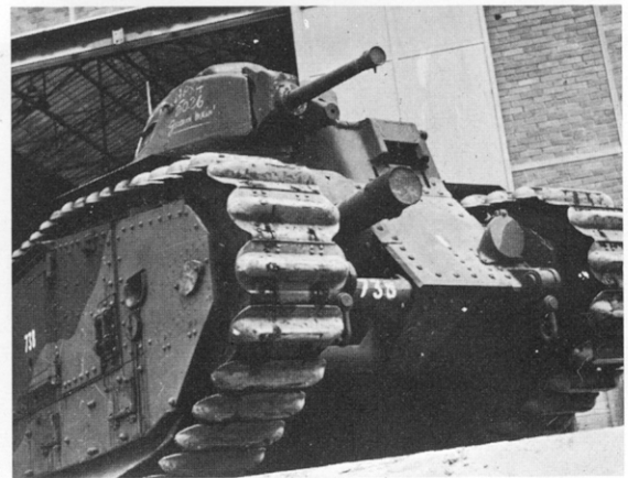
1 Char B1 with short 47mm gun in the APX-1 turret. (I.W.M.)
