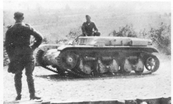
The F.C.M. 36 converted to self-propelled artillery with the standard German 105mm field howitzer. This gun was also mounted on the R 35, the H 39 and the Char B1 bis. (bottom right)
