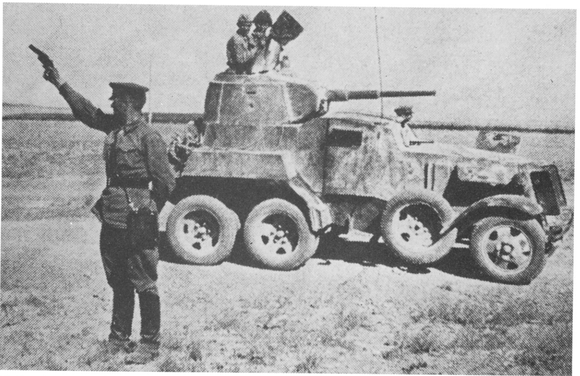
The BA-10 had a turret originally designed for a light tank.
