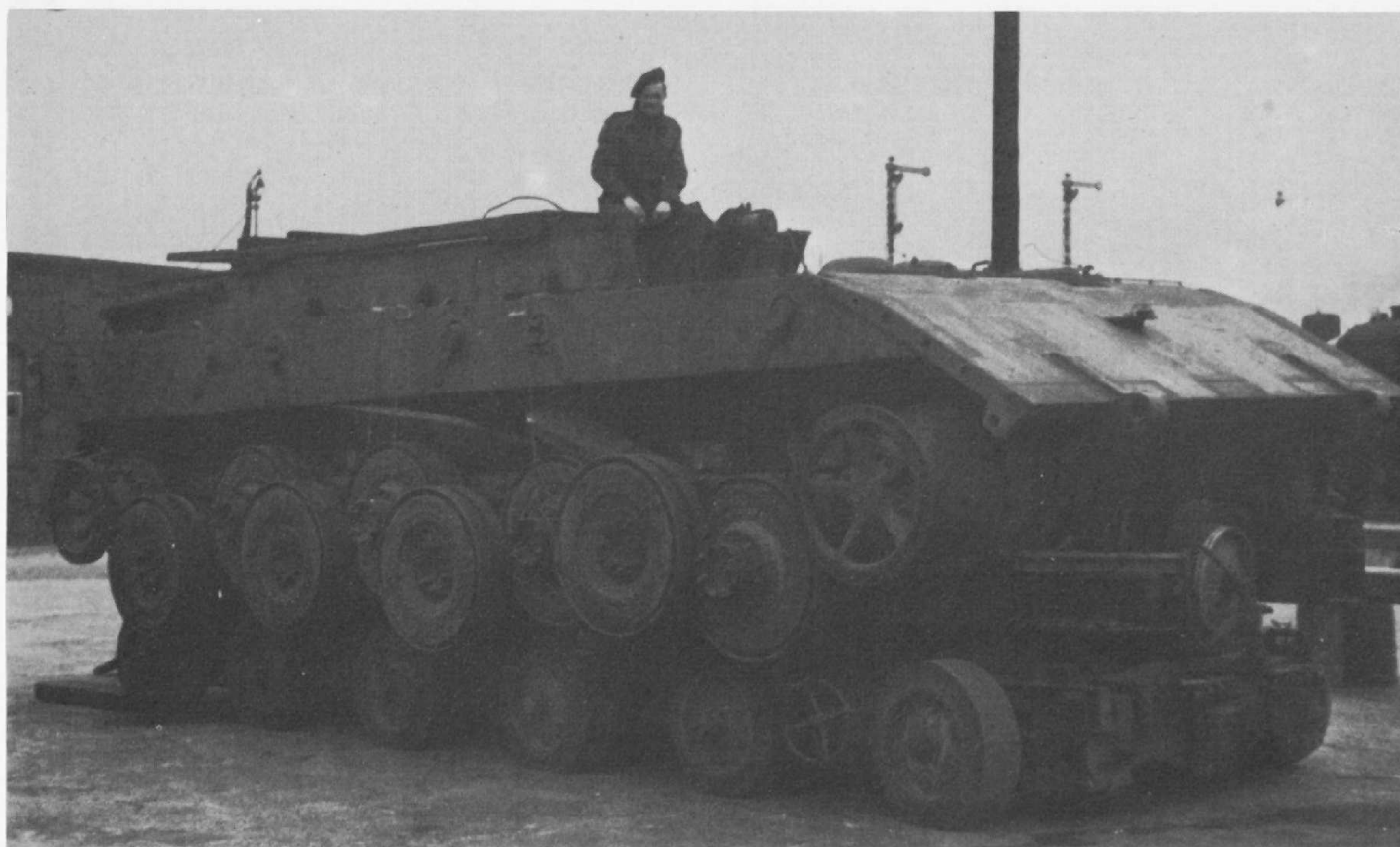
The partially completed prototype of the E-100 has been hoisted on to a low recovery trailer for removal by its captors.
