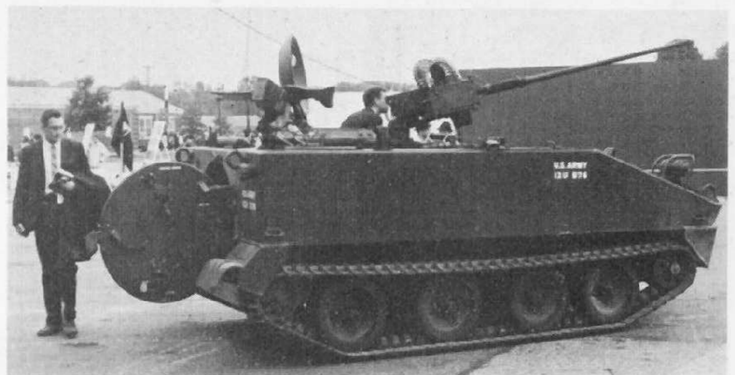
The Product Improved M113A1—no longer a battle taxi but an armoured fighting vehicle. Note the remote-controlled 20mm cannon. (FMC)
