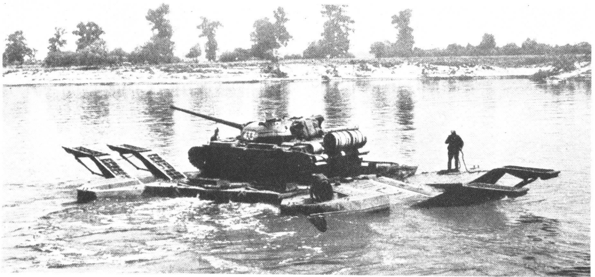
T-54 tank being transported across water by two GSPs joined together.
