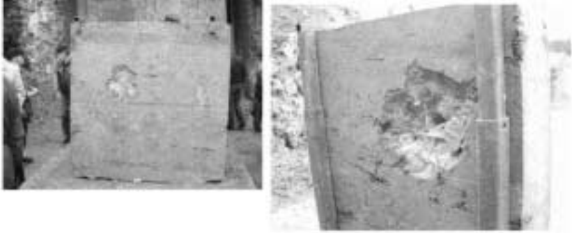
Figure 8. Concrete front and rear side.
